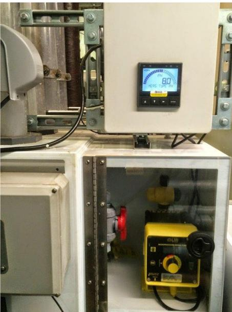
By adjusting the incoming pH to a more neutral range of 7 to 8, the number of regenerations required was reduced from 12 times per year to only 1 to 2 times per year. Also, the total quantity of acids and bases required for neutralization of incoming water supply and regeneration of resins was significantly reduced.
